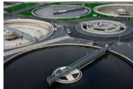
Common Effluent Treatment Plants (CETPs)
